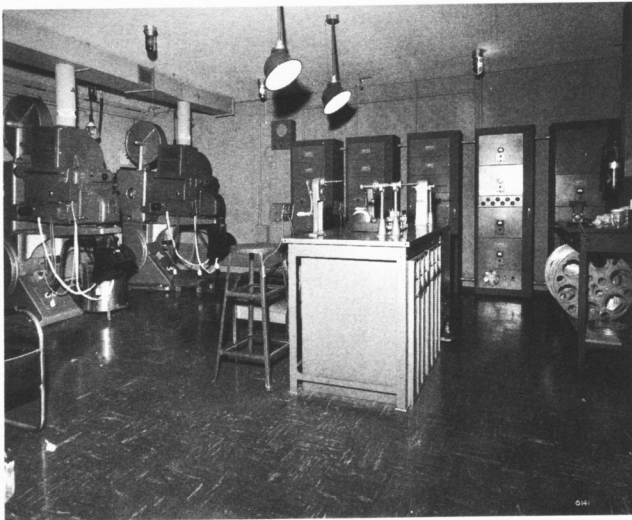
Magnetic reproducing equipment in the motion picture theater. Ampex installation along the far wall (at Warner Theater, New York City) provides six channel stereophonic sound.
